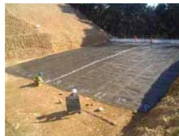
Fig.7. Installation of geogrid layers
